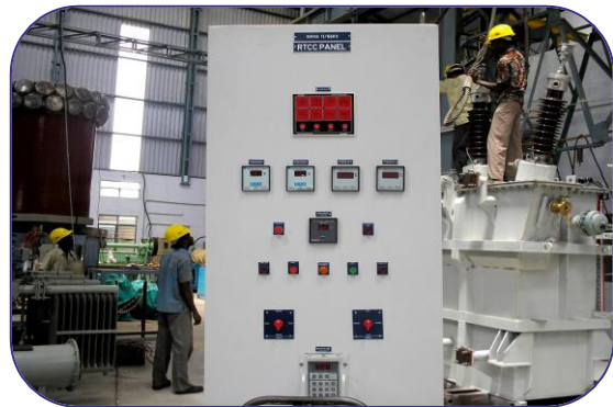
RTCC Panel Assembly
